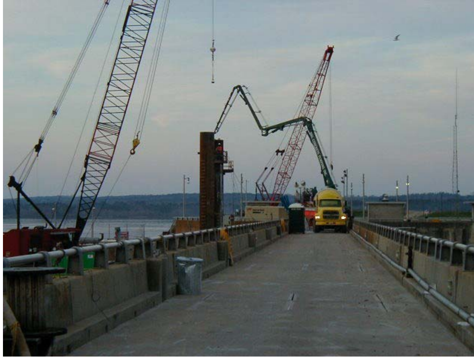
Figure 4.: Rig set up for concrete placement.
