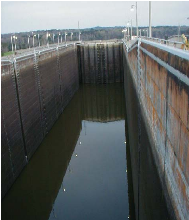
Figure 2.: Looking into a lock at the Walter F. George Dam.
