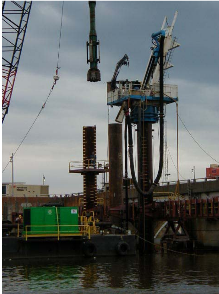
Figure 3.: Setup for pile installation in front of the dam.
